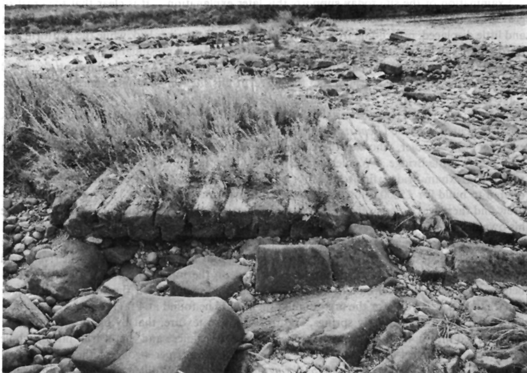
Fig. 4. Platform for one pier of John Gott's bridge, photographed 1974
