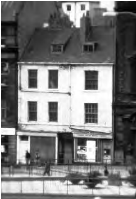
The Golden Tiger public house, photographed in 1977 and subsequently demolished
