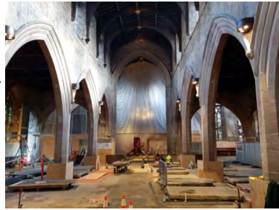
The shrouded Cathedral during its refurbishment, picture David Heslop
