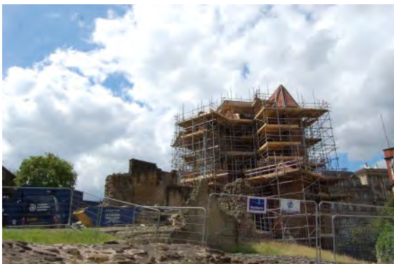
Black Gate under scaffolding.
