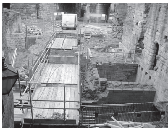
Scaffolding and walkways between the Black Gate and the Castle Keep
