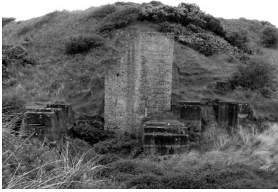
Budle Crushing Plant, picture courtesy Angus Graham
