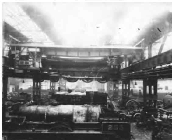
Darlington North Road locomotive works; erecting bay – one of the illustrations from the Darlington volume
