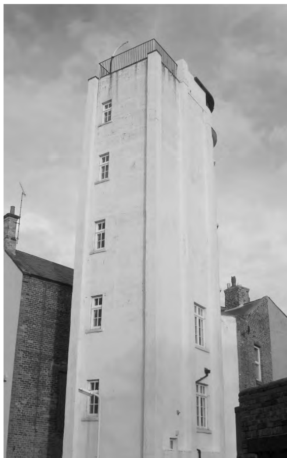
The World War 1 control tower at 47a Percy Gardens, Tynemouth.
